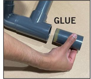
Clean and glue inside the t-piece and outside the 9cm pipe and push together.
