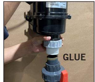
Screw the blower union onto the blower. **HAND TIGHTEN ONLY.** Then clean and glue the outside of the pipe and the inside of the blower union and push together.
