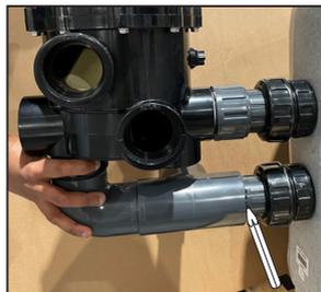
Ensure the multiport valve is horizontal. Mark the bottom pipe if needed so you now how far to push the pipe when you glue it later.
