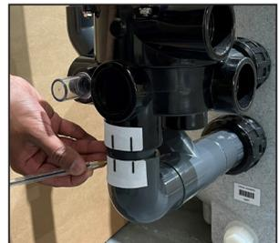
Draw three vertical lines across the two pieces of masking tape. When you glue this later ensure these lines match up.
