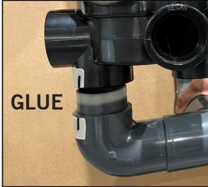
Clean and glue inside the MPV outlet and around the outside of the connector pipe on the elbow and push together. Ensure the lines on the masking tape match up.
