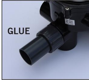
Clean and glue inside the MPV connector and the outside of the 9cm pipe and push together.
