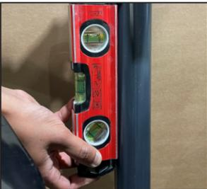
Use a spirit level to check the blower pipe is vertical.
