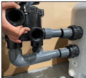
Fit this assembly into the filter inserts until you hit a positive stop. **YOU WILL GLUE THESE CONNECTIONS LATER.**
