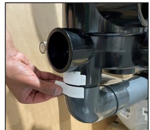
Apply two pieces of masking tape flush to the points where the multiport valve outlet and the connecting pipe join.
