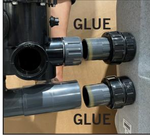
Clean and glue the outside of the inlet and outlet inserts and inside the connectors. Push assembly onto the inserts - matching up to the mark you made earlier if needed.
