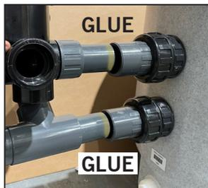
Clean and glue the outside of the inlet and outlet inserts and inside the connectors. Push assembly into the inserts until you hit a positive stop.
