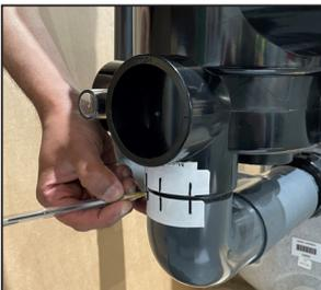
Draw three vertical lines across the two pieces of masking tape. When you glue this later ensure these lines match up.
