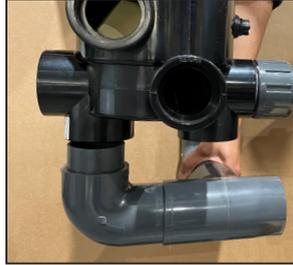
Now take the blower pipework and push the multiport valve outlet onto the upright. **YOU WILL GLUE THIS CONNECTION LATER.**
