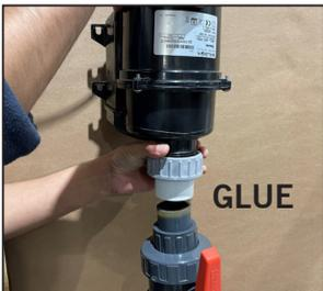
Clean and glue the outside of the pipe and the inside of the blower union and push together.
