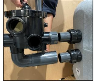
Fit this assembly onto the filter inserts. **YOU WILL GLUE THESE CONNECTIONS LATER.**
