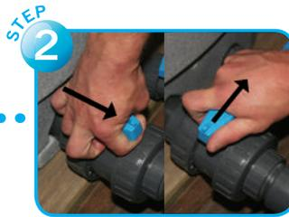
Open the larger waste valve for 2 seconds and then close immediately.
