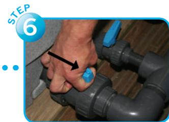
Open the larger waste valve and wait for the inner chamber to empty.
